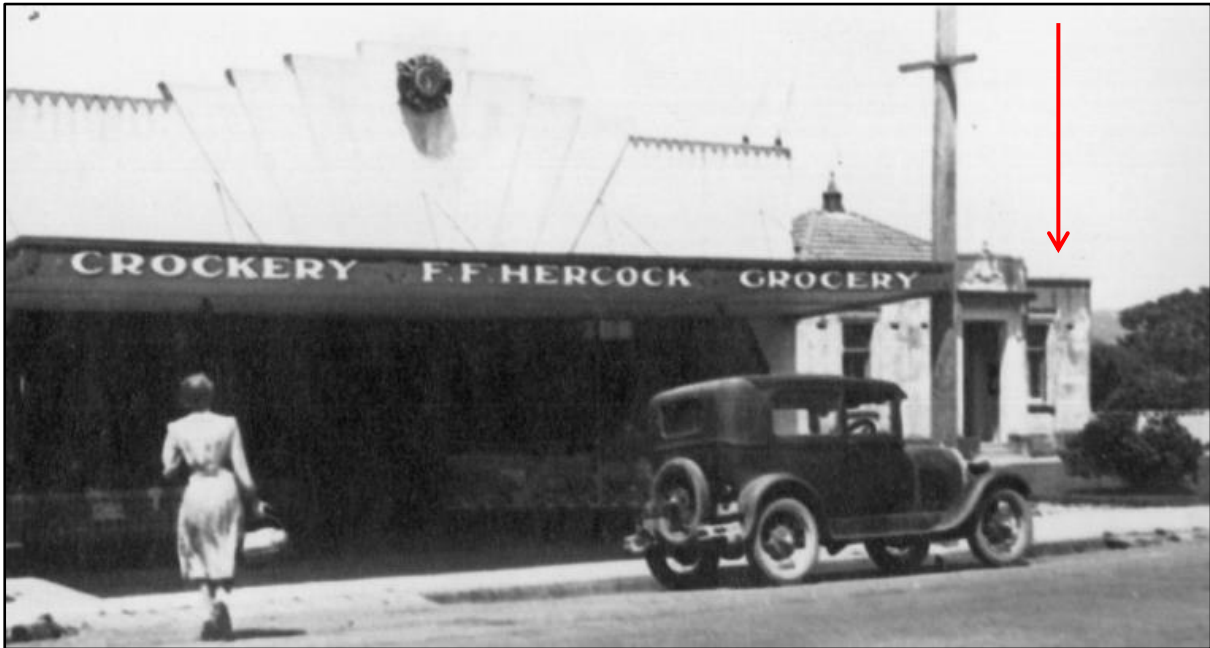
(Reference Upper Hutt City Library Recollect website Main Street Herccock's & Courthouse P2-349-566)
